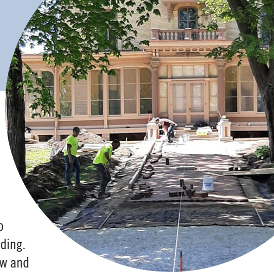
At Villa Louis in Prairie du Chien, workers carefully replaced the walkways leading to and surrounding the historic mansion.
